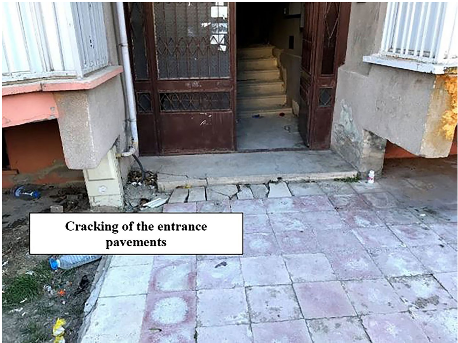
Fig. 31 Cracking of entrance pavement due to seismically-induced lateral displacements observed at the entrance of the of a residential building (38°39'21.9"N 39°09'10.4"E/01.02.2020/14:50)
