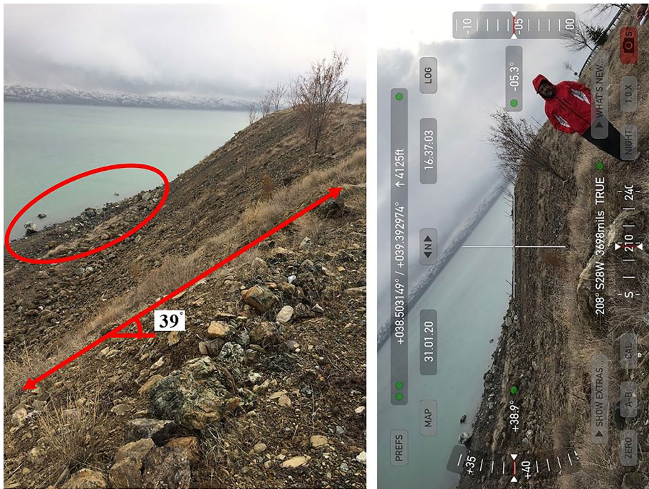
Fig. 18 Rock falls at Site 14 (38°30'11.4"N 39°23'34.9"E/31.01.2020/16:37 & 38°30'11.3"N 39°23'34.7"E/31.01.2020/16:37)
