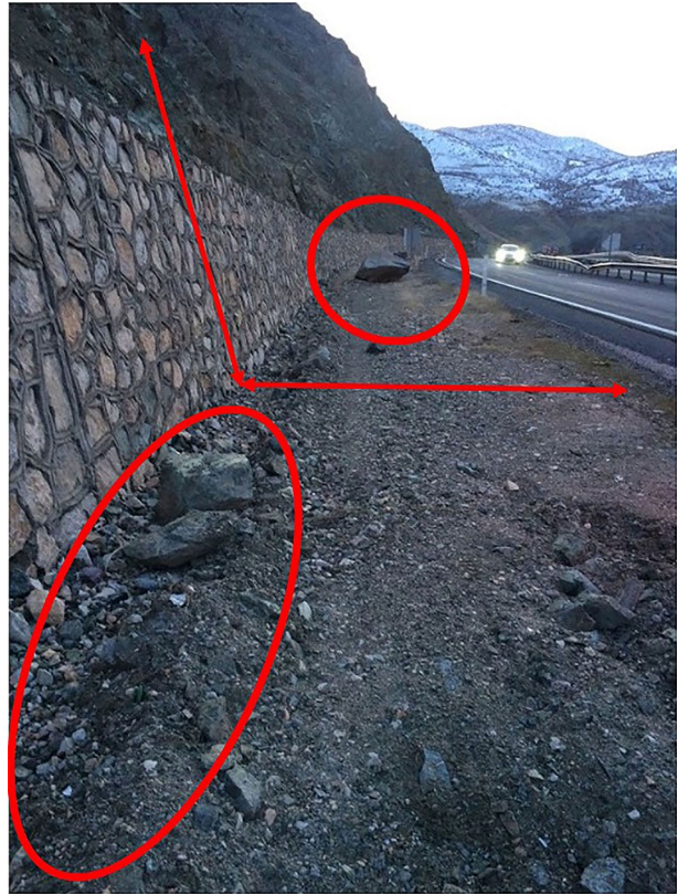
Fig. 19 Fallen rock blocks on the highway bench ( 38^{\circ}26'19.8''\text{N} 38^{\circ}49'38.8''\text{E} /01.02.2020/7:23)
