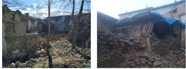
Fig. 29 Damages due to heavy earthen roof at Sivrice township
