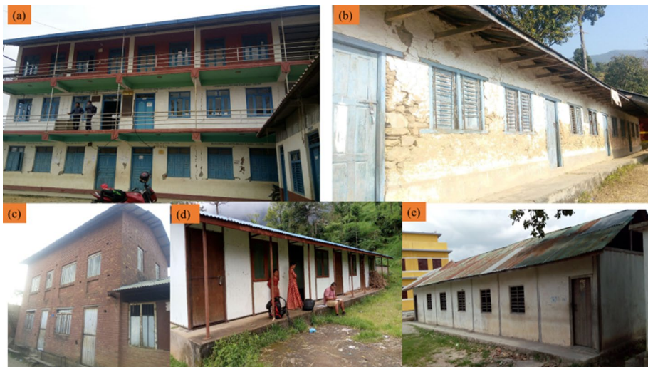
Fig. 1 Building classes considered for development and implementation of the vulnerability assessment framework proposed in this study a reinforced concrete (RC), b stone masonry (LB), c brick masonry (LB), d steel frame, and e timber frame
