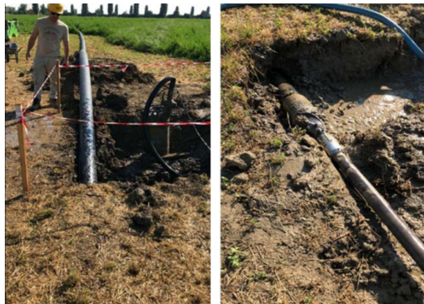
Fig. 24 Final withdrawal of HD well screens, starting point (left) final point (right)
