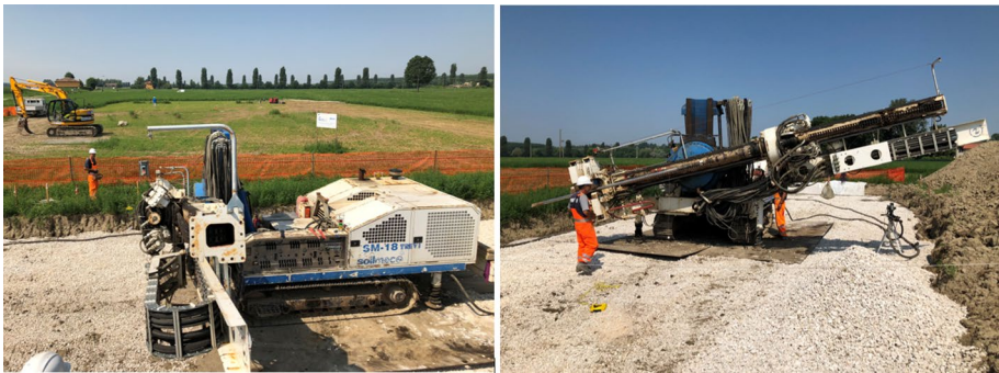
Fig. 22 Drilling equipment set-up during directional drilling activities
