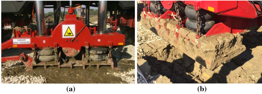
Fig. 29 Test UN_2 in the area 1: (a) picture of sand ejecta during the test and (b) shaker loading plate upon retrieval at the end of the test
