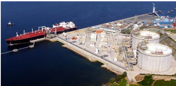
Fig. 1 Overview of refrigerated liquefied gas (RLG) plant
