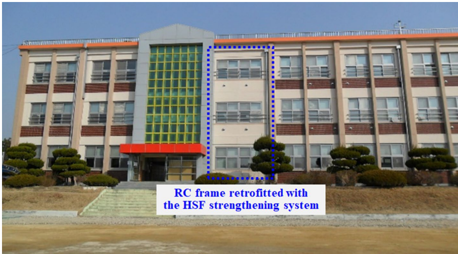
Fig. 1 Post-construction image of the H-section steel frame (HSF) strengthening system
