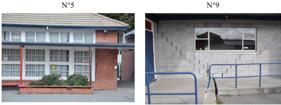
Fig. 21 Buildings C. Brick and Masonry Structures where the lateral stretching was unable to generate a well defined soil or structural mechanism
