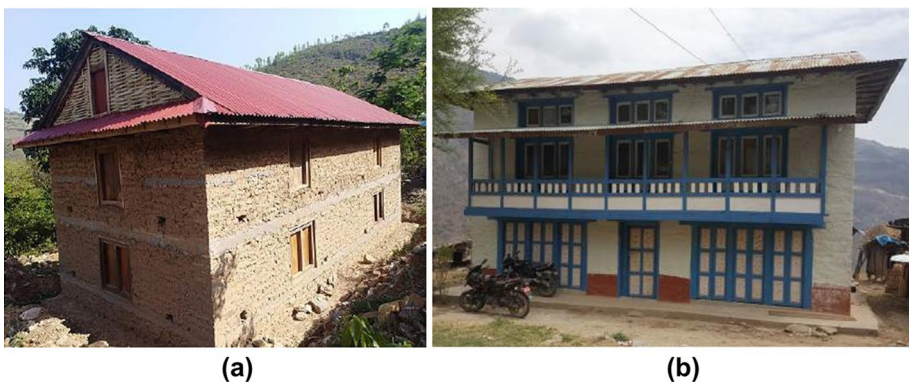
Fig. 5 Photographs of multi-storeyed non-compliant SMM houses built with limited (or without) NRA technical assistance: a photo from Sindhuli and b photo from Solukhumbu (HRRP 2018). In these houses, the seismic bands are not placed at the recommended spacings (Images reproduced with kind permission of HRRP Nepal)
