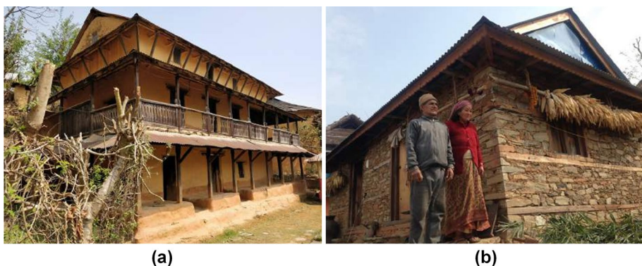
Fig. 6 SMM houses with seismic resistant features of timber elements: a an 80 years old PRE-SMM house in Syangja district that has survived three major earthquakes including the recent 2015 Gorkha earthquake and b a newly built POST-SMM house (HRRP 2018) (Images reproduced with kind permission of HRRP Nepal)
