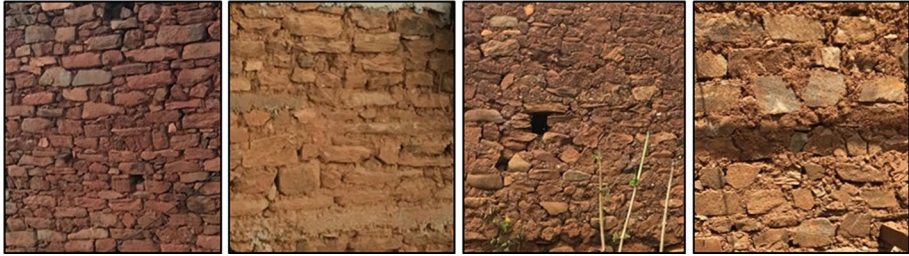
Fig. 7 Masonry bond pattern from 4 different Nepalese SMM buildings
