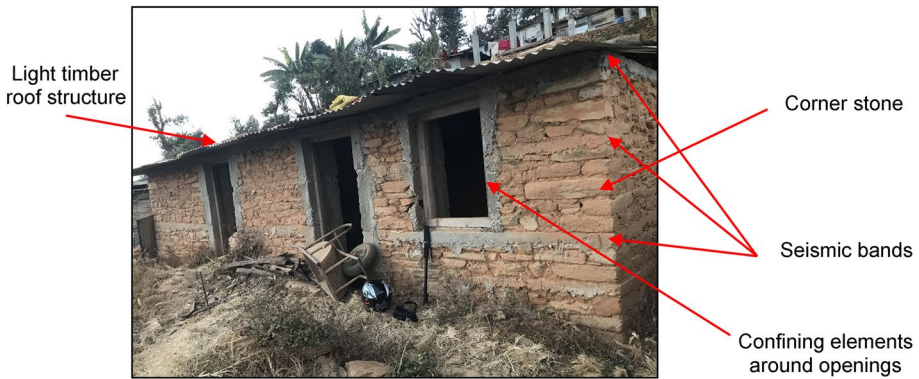
Fig. 9 Construction characteristics of typical POST-SMM buildings (photo from Sindhupalchowk district)
