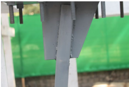
Story Drift = 2.82%: In-plane bending of brace causing slight kink in brace.
