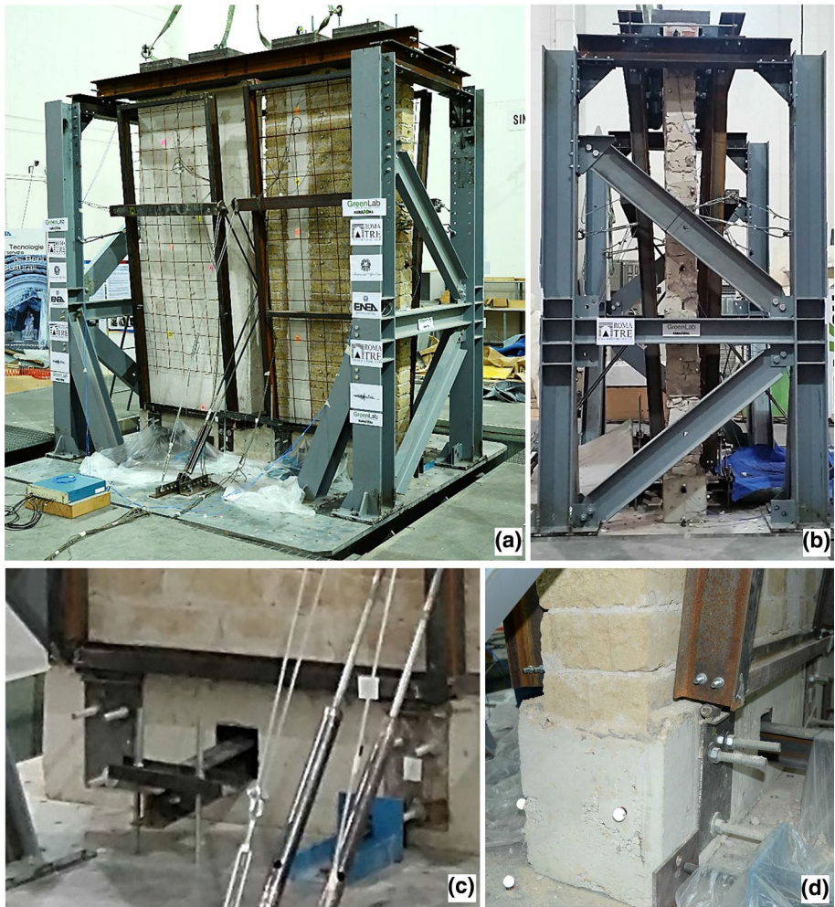
Fig. 1 Perspectival (a) and lateral (b) views of the experimental setup for shake table tests, with details of the anchoring system to the shake table (c) and of the retaining hinged steel frames (d)
