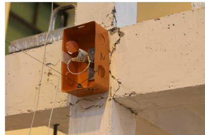
First Story Joint
