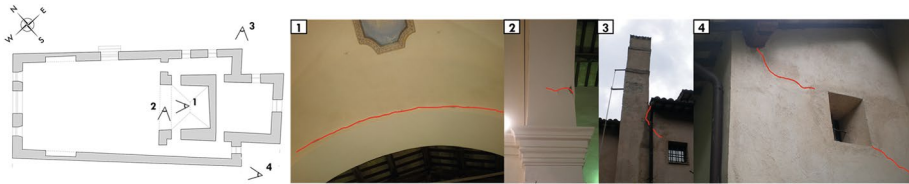
Fig. 11 Damage survey in Madonna of Valcora Sanctuary in Fiuminata after the Central Italy Earthquakes of 2016
