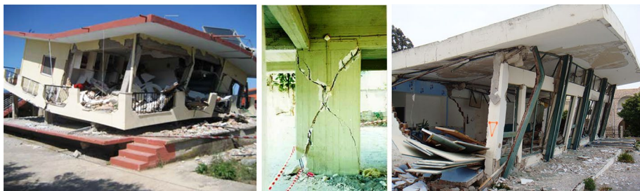
Fig. 1 Brittle failures of R.C. buildings in Greece due to earthquake actions
