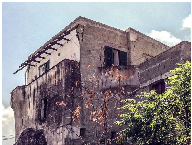
Fig. 21 Undamaged leaf tuff masonry construction with iron tie rods-via provinciale Lacco Fango (Lat: 40.7462–Lon: 13.8899)
