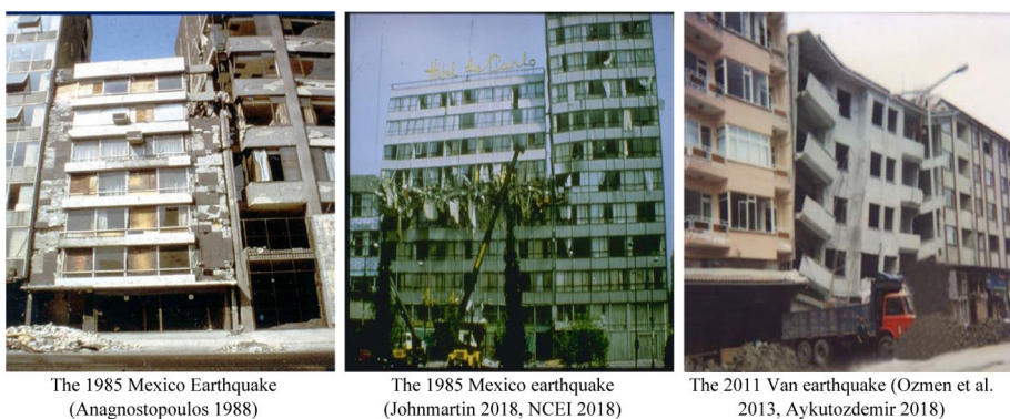
Fig. 1 Pounding damage in adjacent buildings of different heights
