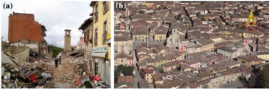
Fig. 2 a Amatrice, after the August 24th event. Extensive damage and collapses in ordinary unreinforced masonry buildings and damage without collapses in tall buildings: six-storey reinforced concrete building, on the left, and Clock Tower from Corso Umberto I. b Part of the historical centre of Norcia after the October 30th event in the snapshot of a movie released by the Corps of Firefighters ( www.vigilfuoco.tv ). Limited damage to ordinary unreinforced masonry buildings and extensive collapses to churches: (1) Santa Rita, (2) San Francesco, (3) Santa Maria Argentea, (4) San Benedetto and (5) San Filippo
