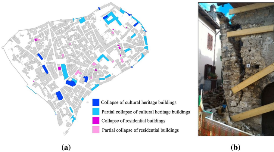
Fig. 5 Identification of collapse in residential and cultural heritage buildings (a); collapse of a masonry unit (b)
