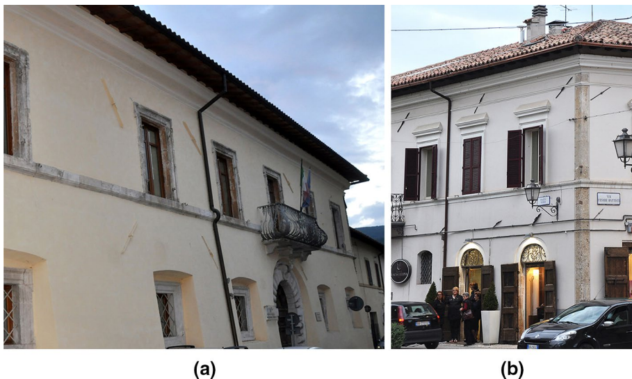
Fig. 3 Norcia. Two-storey buildings, tapered wall thickness, systematic use of tie rods. a Via Cavour; b Piazza Giuseppe Verdi
