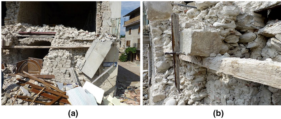
Fig. 7 Iron wall anchor of timber tie, Amatrice, via Roma. a General view; b Close up of a wall anchor
