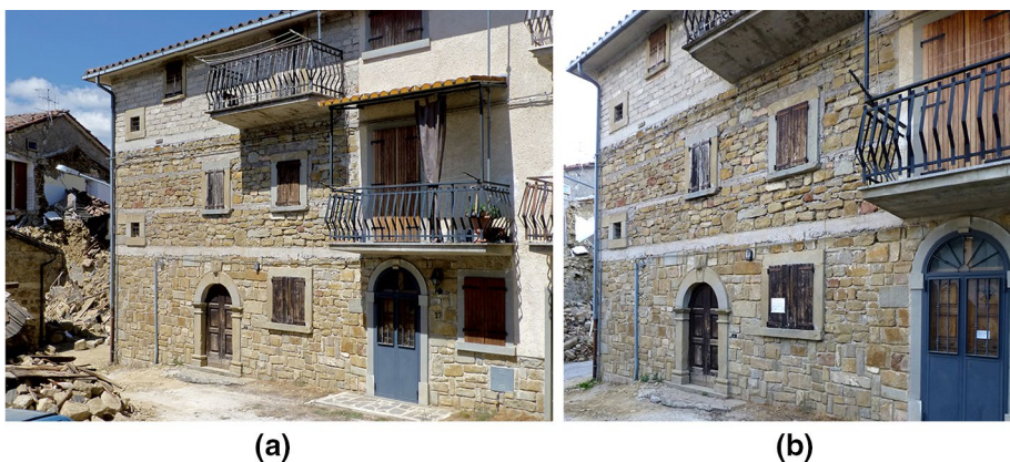
Fig. 17 Demolished and rebuilt natural stone masonry, resorting to modern mortar and ring beams. Amatrice, San Capone. a Post 24th August; b post 30th October
