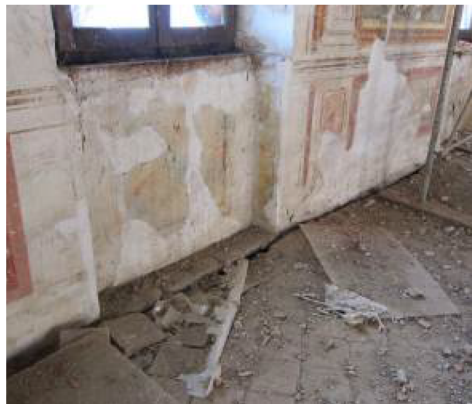
Fig. 1 Typical failure mechanism involving the overturning of the perimeter walls: a overturning of the façade and lateral walls in S. Agostino Church (as it was after the first shock of August 2016); b detachment of a perimeter wall in Villa Galvagnina hit by the Emilia earthquake in 2012
