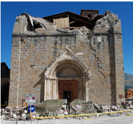
Fig. 1 Typical failure mechanism involving the overturning of the perimeter walls: a overturning of the façade and lateral walls in S. Agostino Church (as it was after the first shock of August 2016); b detachment of a perimeter wall in Villa Galvagnina hit by the Emilia earthquake in 2012
