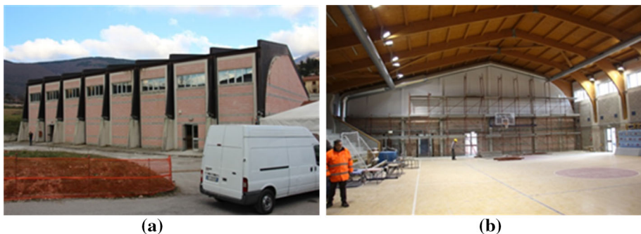
Fig. 6 The gym structure: external (a) and internal view (b)
