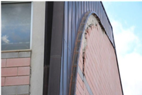
Fig. 7 Separation of the external layer of infill panels
