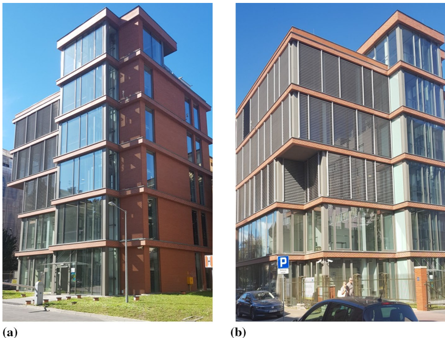
Fig. 1 View of the building: a north-east elevation, b south-east elevation
