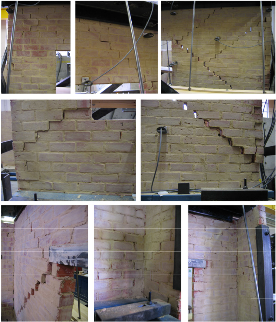
Fig. 13 Wall D3 at the conclusion of testing
