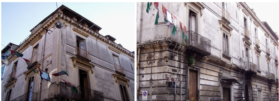
Fig. 3 External views of the “Pelella Palace”
