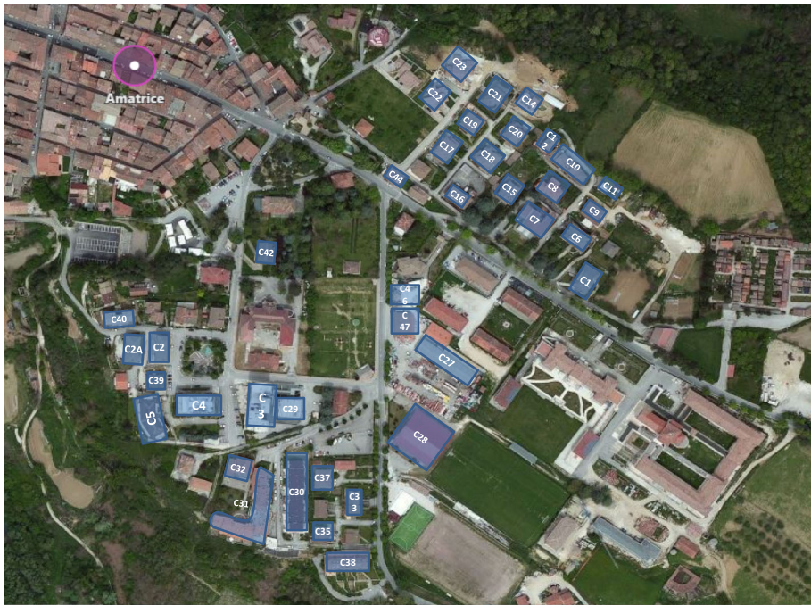
Fig. 4 RC buildings surveyed in the town of Amatrice. RC buildings are indicated by a “C” prefix and are progressively numbered from C1 to C37
