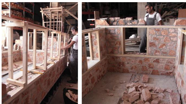
Fig. 5 Timber ties and timber frames around openings
