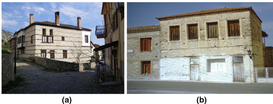
Fig. 1 a, b Typical timber reinforced buildings in Greece
