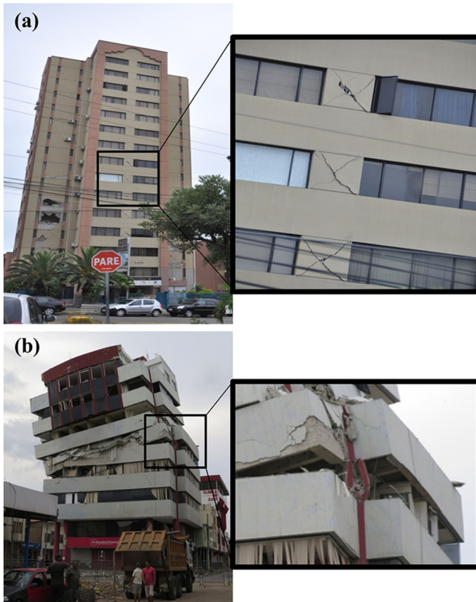
Fig. 11 15-storey RC building in Manta (a) and partial collapse of 9-storey RC building in Portoviejo (b)
