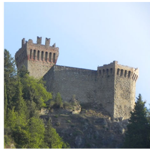
(c) Arquata del Tronto Castle, Central Italy 2016
