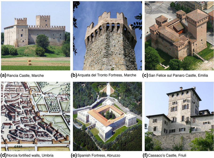
Fig. 2 Typical features of Italian fortified architectures from different historical periods: a crenelated parapet with merlons; b machicolations; c an aerial view of a typical fifteenth century castle; d a fortified citadel; e a fortress with bastions, introduced to withstand attacks with firearms, from the sixteenth century; f a medieval castle transformed into residential palace
