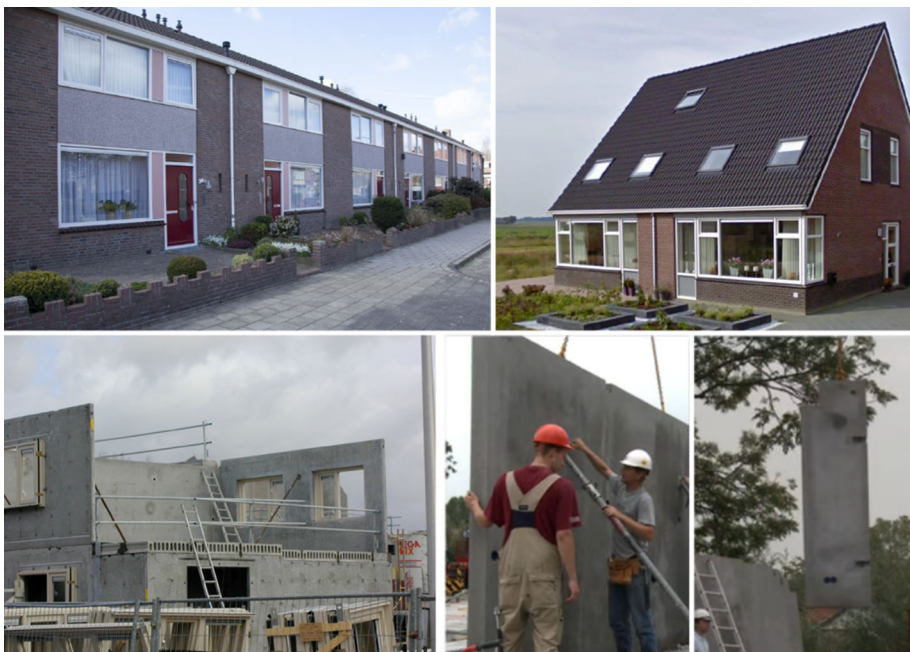
Fig. 1 Examples of typical multi-unit precast RC houses and key details of the construction process
