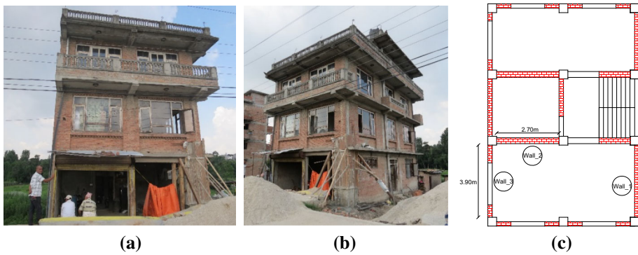
Fig. 16 General view of the NE3D building, a front view, b lateral view and c building plant and localization of the IM walls under study
