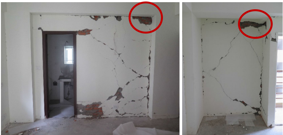
Fig. 12 Stress accumulation in the top and bottom corners observed in interior partition walls of a high-rise residential building
