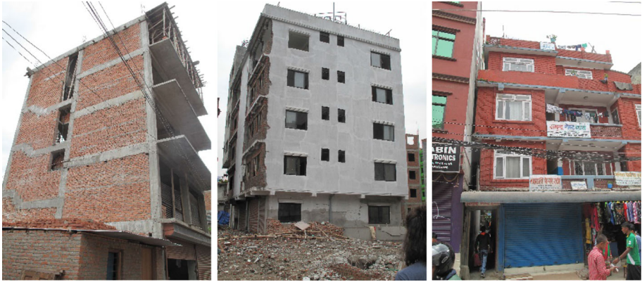
Fig. 8 IM walls typologies most common in Nepal
