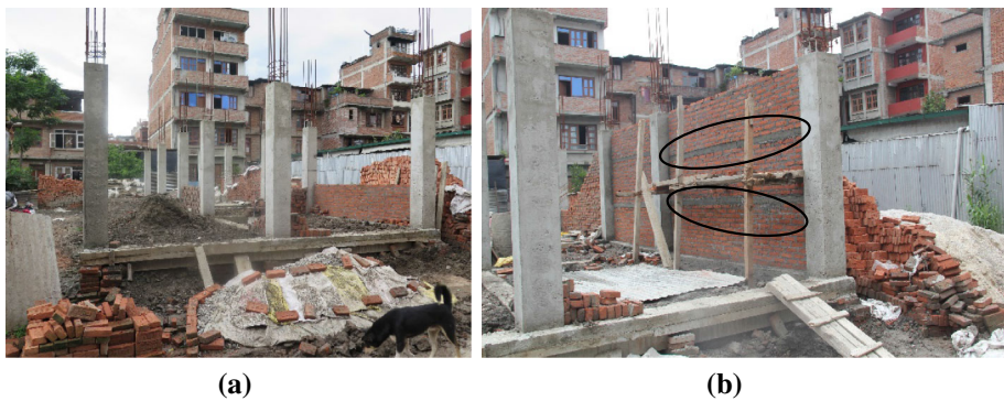
Fig. 5 Typical IM walls construction process in Nepal
