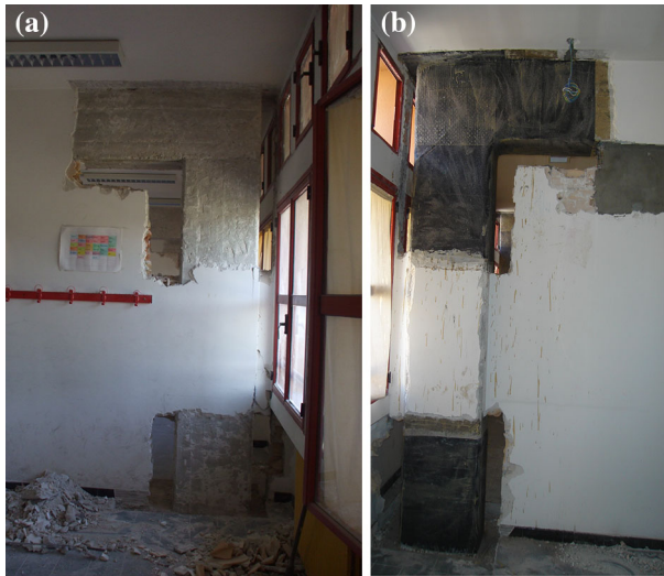
Fig. 11 FRP-based interventions to increase the joint shear capacity of unconfined joints (a) and the deformation capacity in the critical zones of columns (b)
