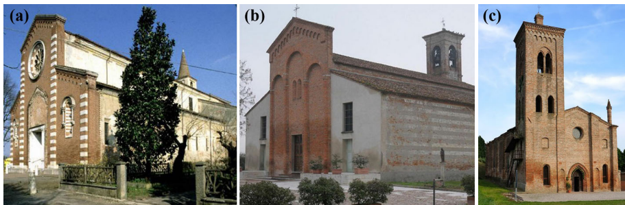
Fig. 1 General view of the three churches under study: a San Benedetto Abate church in Gonzaga, b San Fiorentino Martire church in Nuvolato, c Santa Maria Assunta church in Felonica
