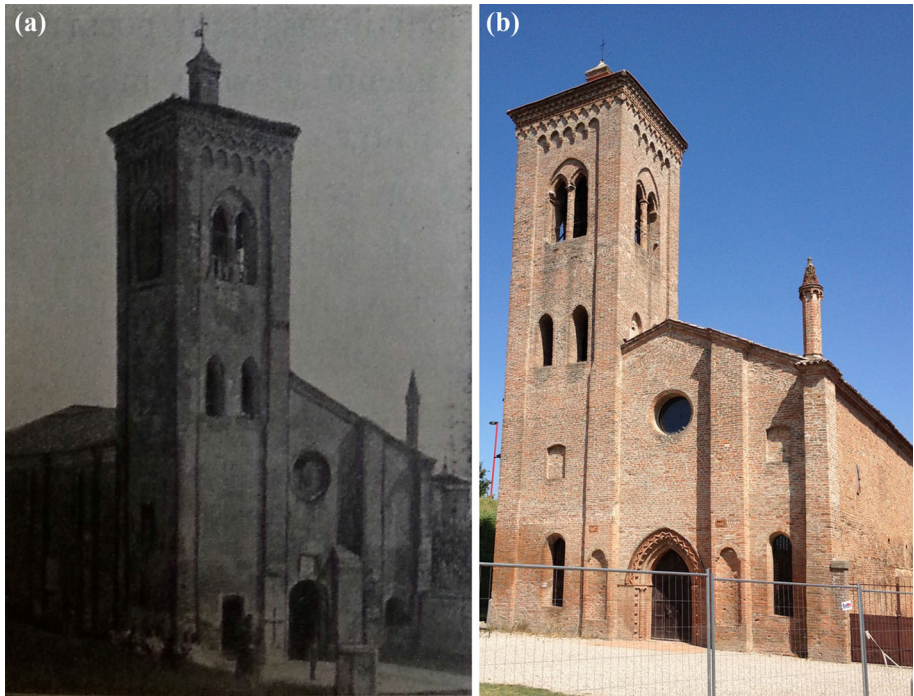
Fig. 4 Santa Maria Assunta church: the external view a before and b after the interventions performed between 1915 and 1920 by Aldo Andreani
