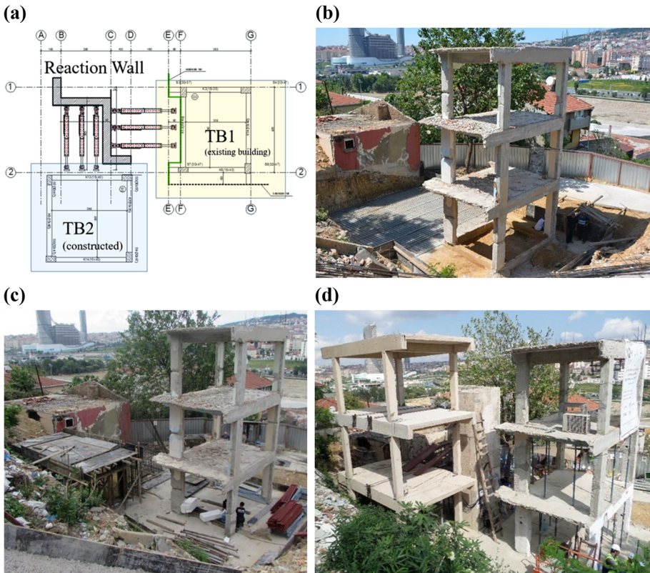
Fig. 2 a Layout of the test site and b–d stages of site preparation
