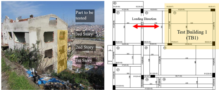
Fig. 1 General view of the test site and plan of the existing building
