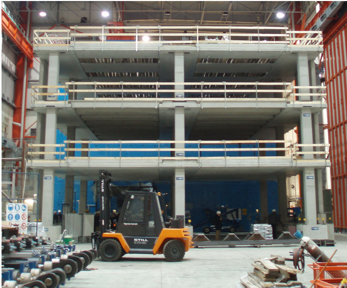
Fig. 14 Precast structure full scale 3-storey prototype assembled at the ELSA laboratory of the JRC of the EU in Ispra (Italy)
