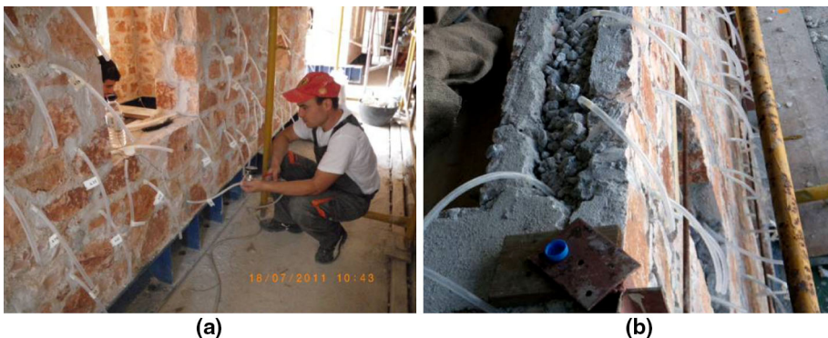
Fig. 5 a–b Grouting of three-leaf masonry walls
