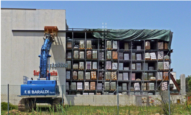
Fig. 2 Warehouse in Medolla
