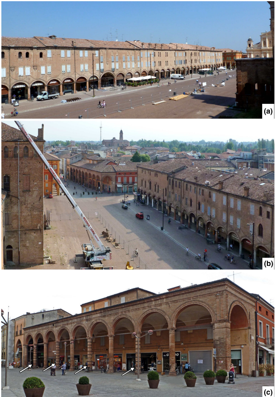
Fig. 13 a The Portico Lungo in Piazza Martiri seen from the south; b an overview of the Piazza Martiri arcades from the north; c Portici del Grano in Via Alberto Pio : arrows indicate the columns that have been consolidated
