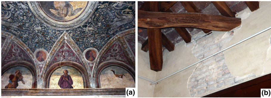
Fig. 17 Palazzo dei Pio — a frescoes with cracks. b extraction of a roof beam on the upper level of Torre del Passerino
