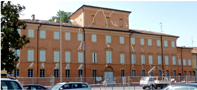
Fig. 5 Palazzo Sartoretti —the old Town Hall (the main façade heavily damaged)
