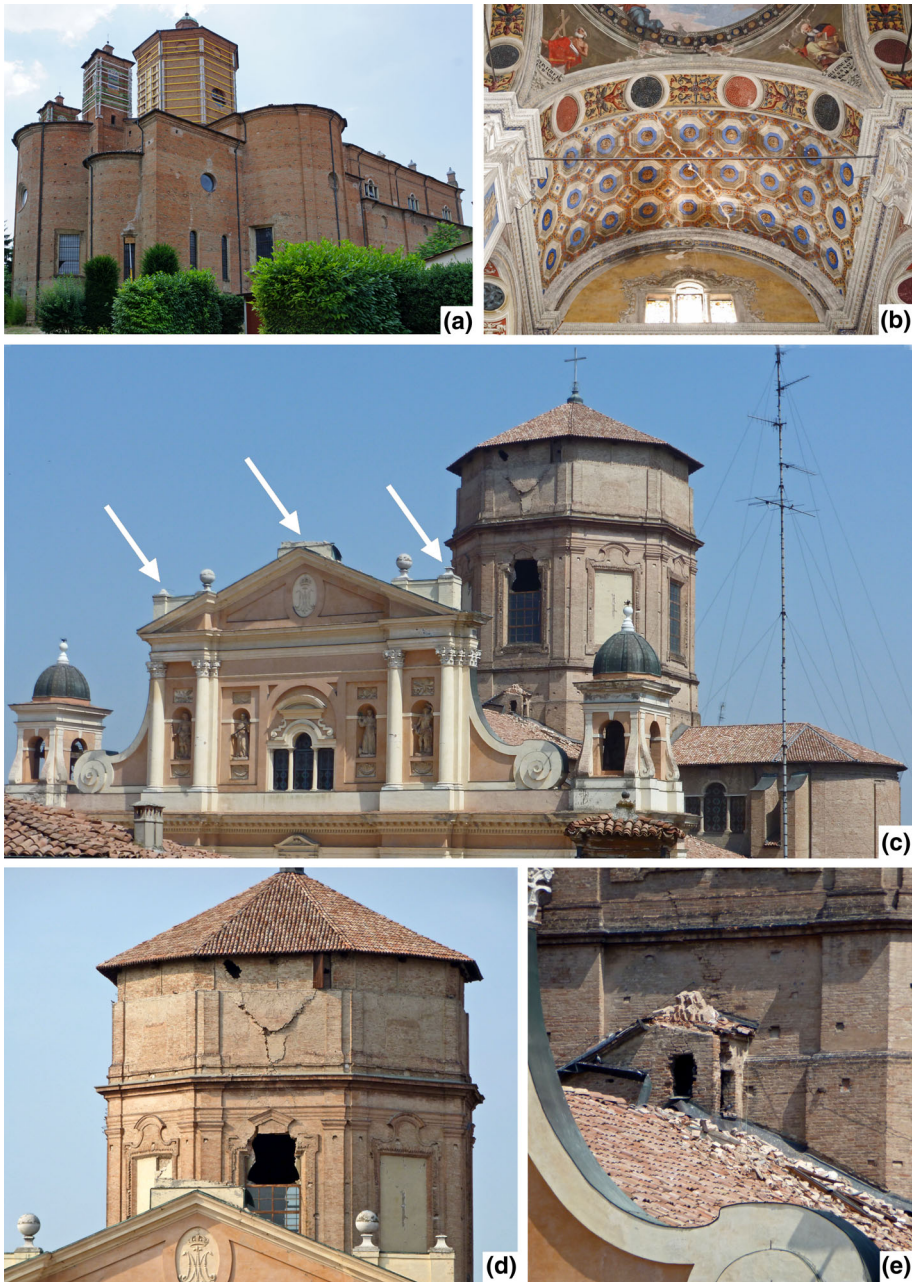
Fig. 15 a Rear side of San Nicolò church; b new and existing damage in the barrel vault in San Nicolò ; c–e cathedral of Assunta : fallen ornaments and damage to roof and dome
