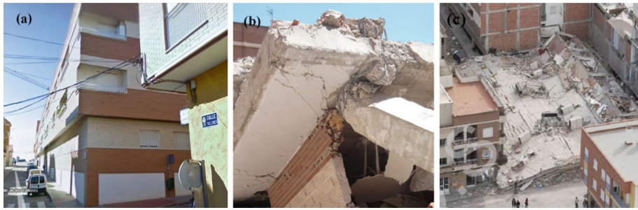
Fig. 10 The only building collapsed due to the Lorca earthquake, before (Google Street View) (a) and after the event (b, c). Photograph c adapted from Regalado and Lloret (2011)
