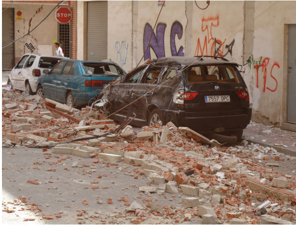
Fig. 1 Street covered with rubble of damaged buildings
