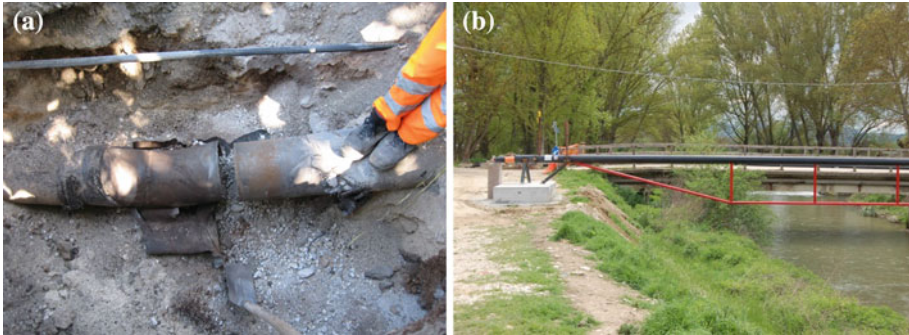
Fig. 6 Damage to gas pipes following the L’Aquila earthquake: a gas welded joint of a LP steel pipe pulled apart in Paganica (AQ); b gas pipe connected to a damaged bridge in Onna (AQ) replaced with a stand-alone pipe (photos courtesy of ENEL Rete Gas)
