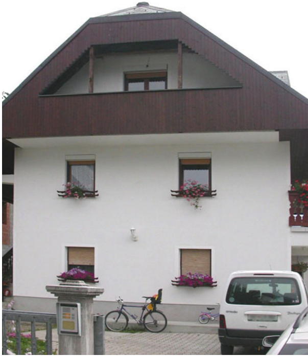
Fig. 1 Confined AAC masonry house in Bovec, Slovenia, resisted M = 4.7 earthquake in 2004 (PGA 0.47 g in the vicinity) without damage (photo by U. Klemen)
