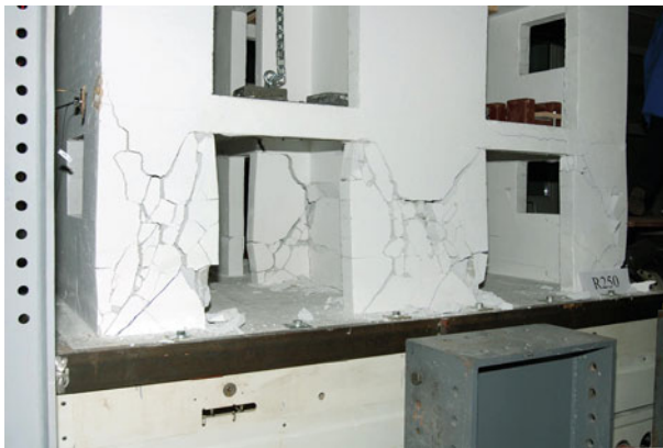
Fig. 22 Damage to the walls in the ground floor of model M2 at ultimate state
