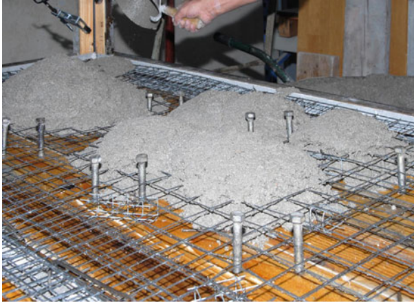
Fig. 12 Reinforcement of monolithic r.c. slabs
