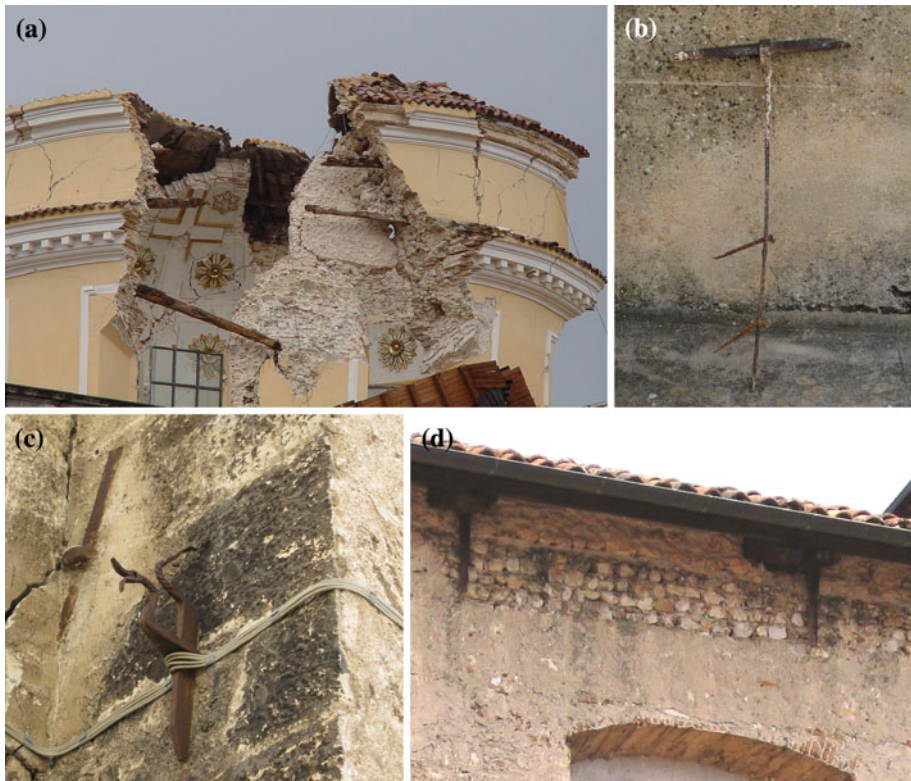
Fig. 6 Some examples of “wooden ties” and connections: a “wooden ties” at different levels of the dome of Santa Maria del Suffragio church in L’Aquila; b the terminal connection elements, taken from the debris: the key and the steel plate (with two nails); c the external key; d and external wooden key for the connection of the trusses in Santa Maria del Carmine church in L’Aquila
