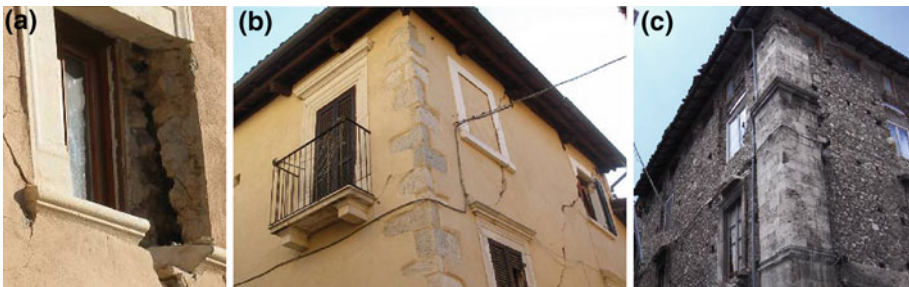
Fig. 5 Examples of a 'muratura a sacco' and of b–c stone quoins. The photo on the right is of a building of the XIV century in which two storeys have been added under and above the original roof line
