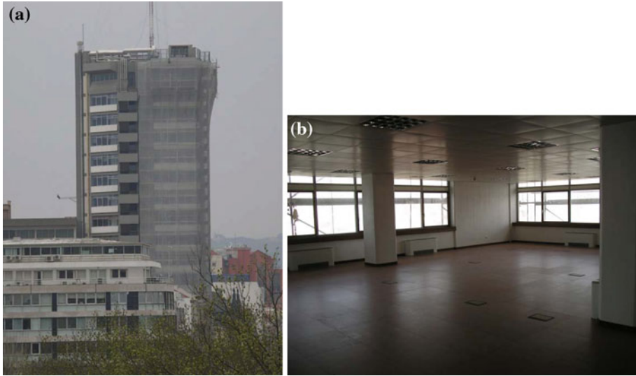
Fig. 9 Recent MRF+SW structures without interior infill brick walls ( open spaces ): a exterior view; b interior view
