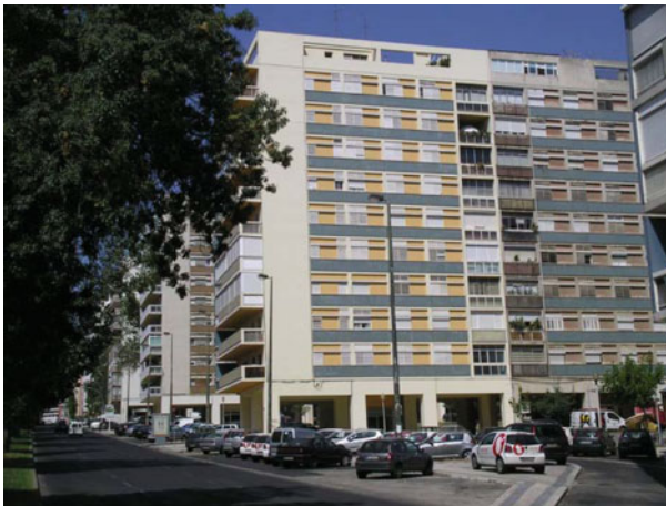
Fig. 10 Typical soft-storeys buildings in the 1960s (“pilotis”)
