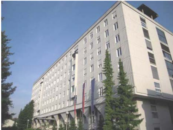
Fig. 2 The investigated multi-storey RC building
