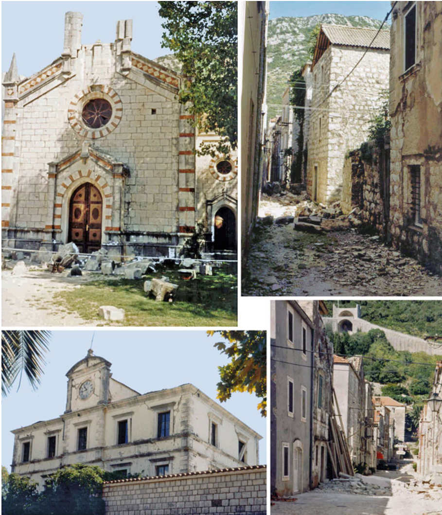
Fig. 8 Damage to buildings caused by the Ston-Slano earthquake of 1996. Top left St. Blasius church. Bottom left Ston Town Hall. Top right W–E running street. Bottom right S–N running street with the Stoviš tower in the background. Photographs by M. Herak, 1996
