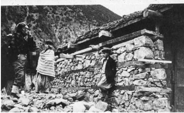
Fig. 50 Traditional dwelling in North West Frontier Province, Pakistan, with timber-laced walls and independently supported roofs. Survivor of the 1974 Pattan earthquake (Source: Ambraseys et al. 1975 )
