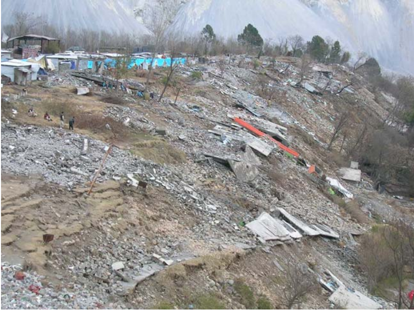
Fig. 51 Kashmir earthquake of 2005. Complete failure of concrete block masonry dwellings, Muzaffarabad (Authors photo)
