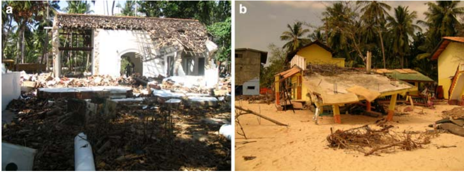
Fig. 37 The 26 December 04 tsunami: typical building damage at Unawatuna, Sri Lanka where the tsunami run-up height was about 5 m in (a) masonry and (b) reinforced concrete structures (Courtesy of the Earthquake Engineering Field Investigation Team EEFIT, UK)
