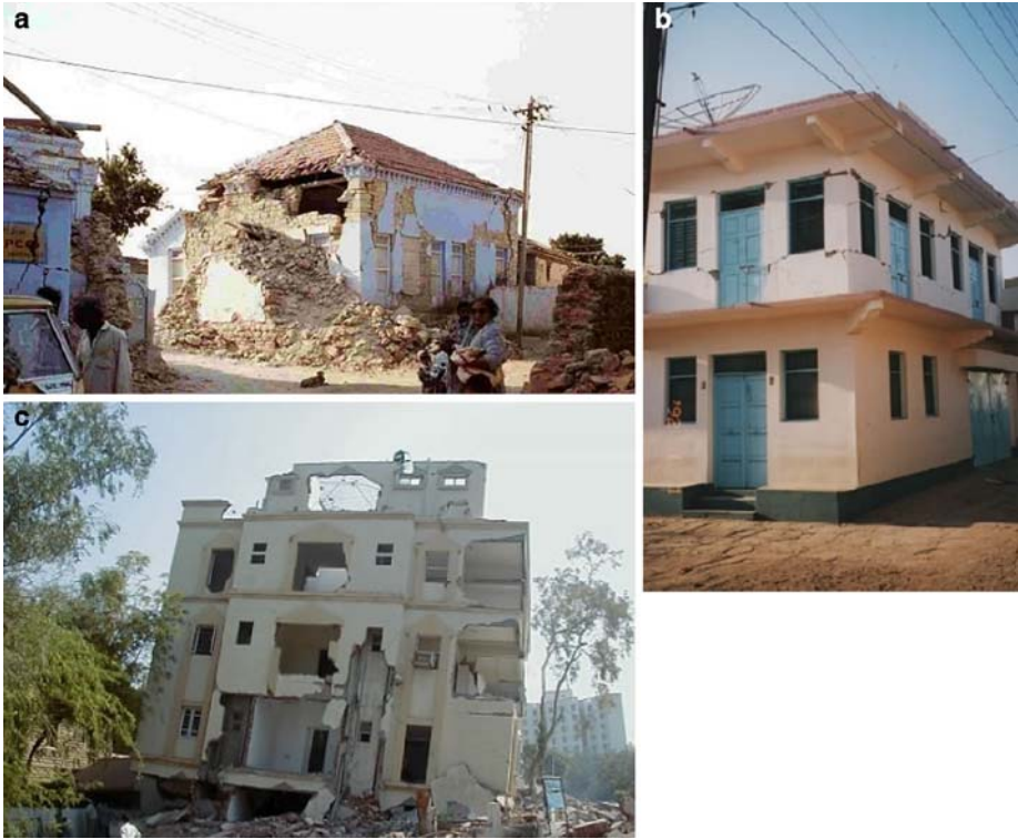
Fig. 29 Masonry and reinforced concrete building types in the Katchchh District ( a, b ) and typical damage patterns. Notice ground floor failure of the reinforced concrete building ( c ) (author's photos)
