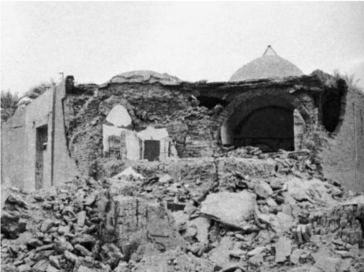
Fig. 33 Failure of adobe structure in Bam earthquake (source: World Housing Encyclopedia, Reproduced by permission of Earthquake Engineering Research Institute)
