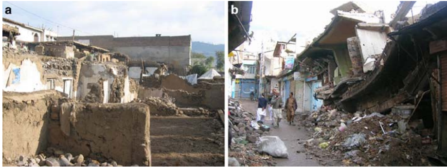
Fig. 39 Traditional masonry construction (a), and damage to reinforced concrete construction (b), Kashmir earthquake (Photos courtesy of Emily So (a) and author (b))
