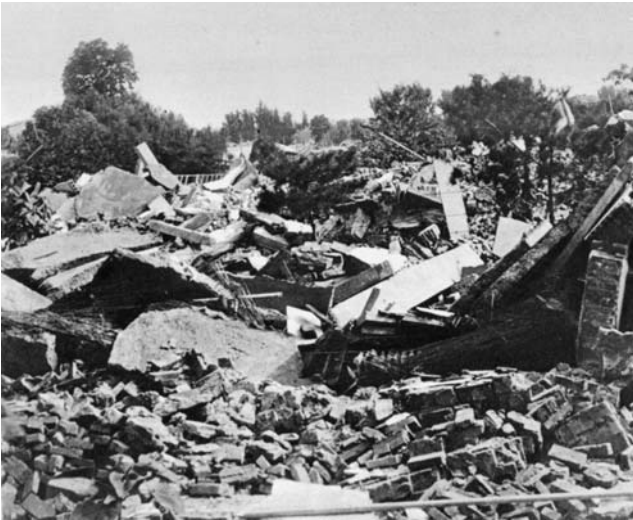
Fig. 16 The huge death toll was mainly due to the total collapse of many brick masonry apartment buildings such as these (source: China Academy of Building Research 1986 )
