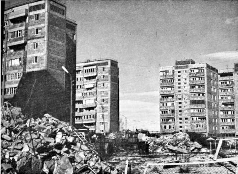
Fig. 19 Spitak earthquake of 7 December 1988. Nine-storey precast concrete frame buildings in Leninakan. The ones standing are severely damaged. Many collapsed completely (source: Wyllie and Filson 1989 , Reproduced permission of Earthquake Engineering Research Institute)
