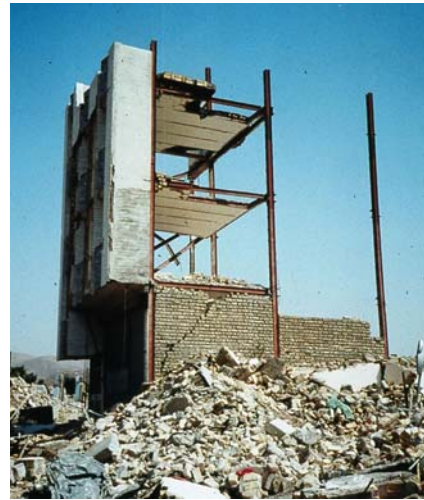
Fig. 23 The Manjil Iran earthquake of 21 June 1990. Failure of infilled steel frame building (source: EEFIT Image Database, Courtesy Earthquake Engineering Field Investigation Team (EEFIT) UK)
