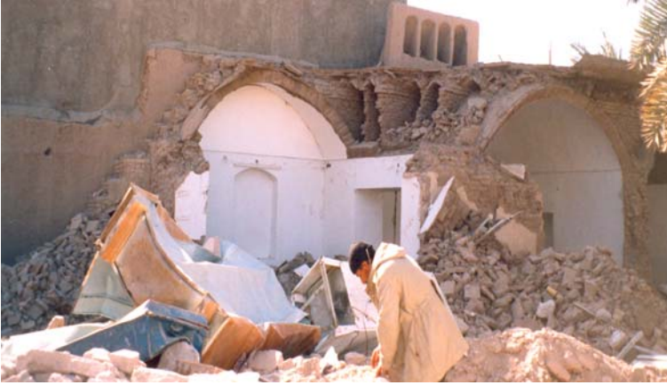
Fig. 32 Bam earthquake: collapse of typical adobe dwelling with vaulted roof (photo courtesy of Jubin Motamed)
