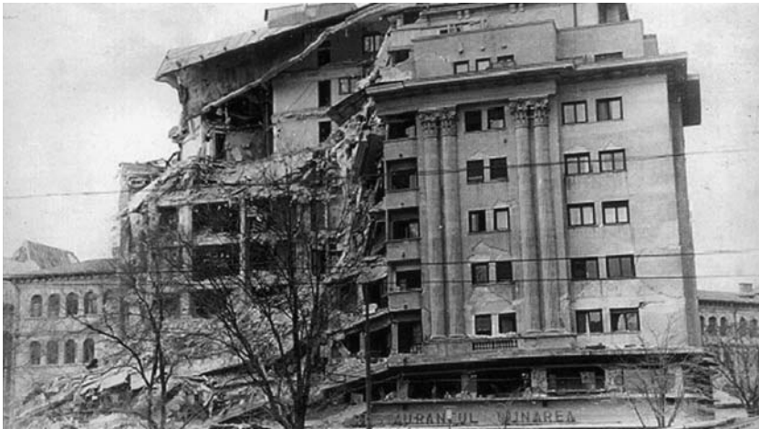
Fig. 44 Bucharest: apartment block damaged by the 1977 earthquake; many such apartment blocks were poorly repaired after the earthquake and upgrading is now in progress (Source: INCERC, Romania)
