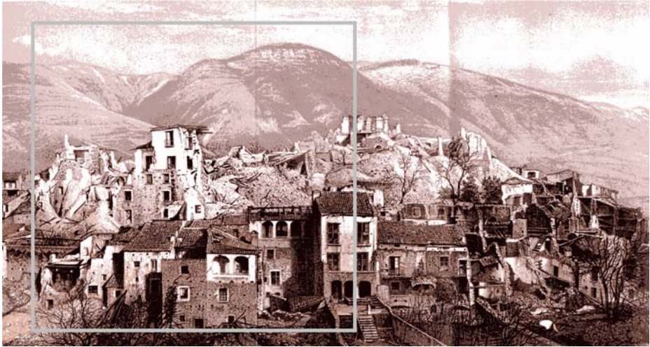
Fig. 1 The damage to Polla, in Irpinia, in the 1857 earthquake (from frontispiece of Mallet 1862)
