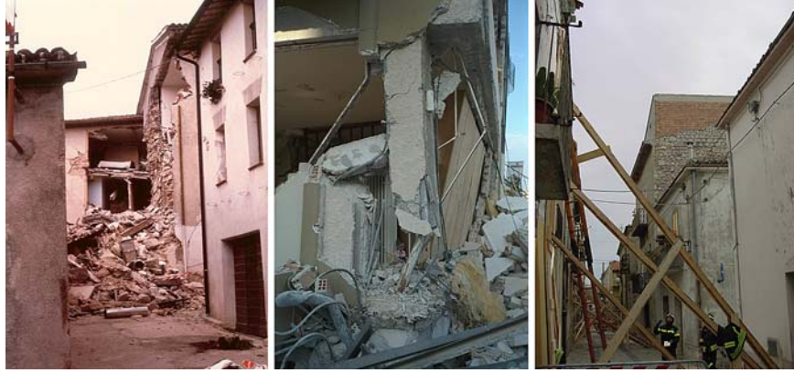
Figure 1. Examples of road blockage due to (i) out of plane wall overturning in masonry buildings (Marche 1997, Italy), blockage type o, (ii) heavy damage to RC concrete building (Athens 1999, Greece), blockage type c, and (iii) short-term countermeasures in masonry building (Molise 2002, Italy), blockage type p.
