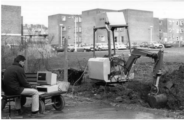
Fig. 1 Robot excavator under ‘training’
