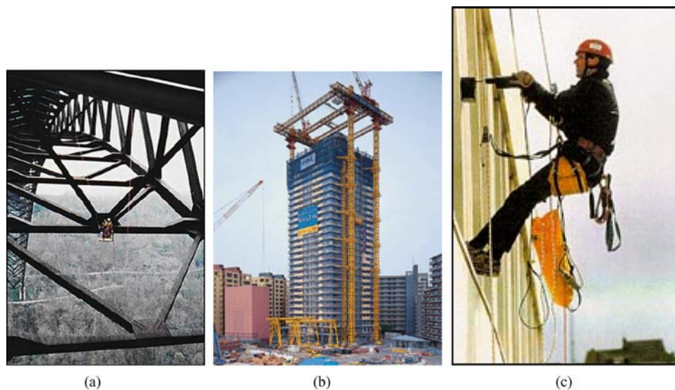
Figure 1. Different climbing environments: (a) steel-based bridge, (b) building steel-based skeleton, and (c) its manual inspection.
