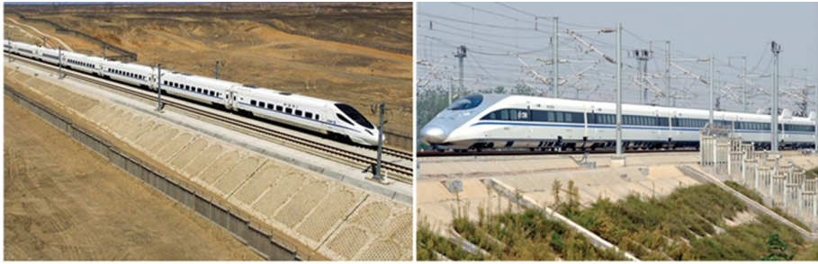
Fig. 1 The embankment along a railway line
