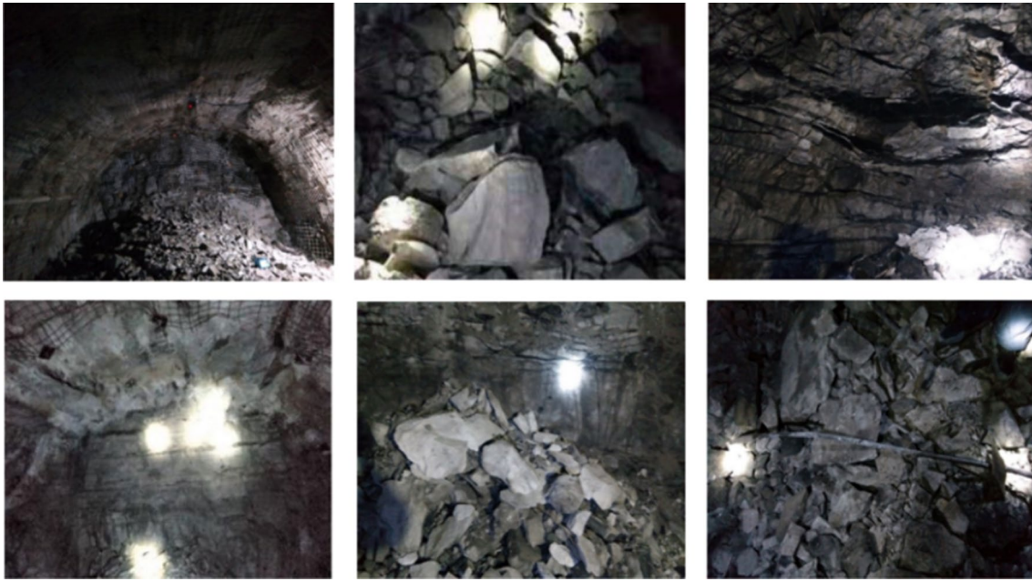
Fig. 3 Practical problems of on-site blasting in roadway excavation
